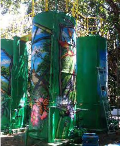
Figura 15 – Reator UASB ETE Iparana
