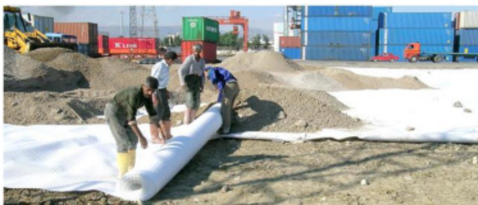
FIGURA 3.23 - Instalação de Geocomposto no Porto de Mersin (European Association of Geosynthetic product Manufacturers).
