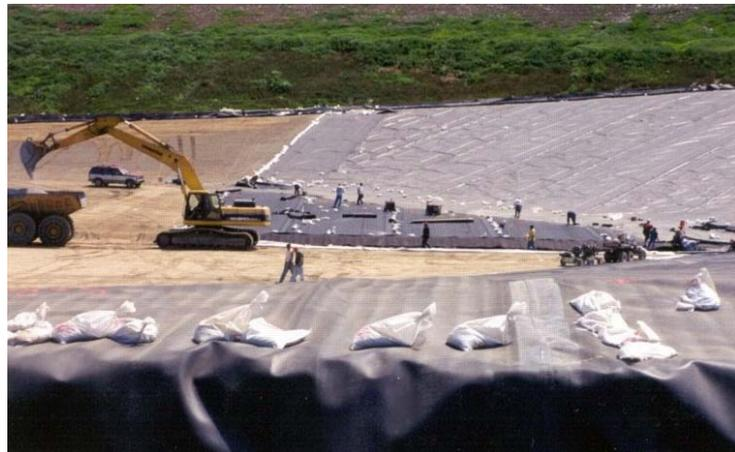
**Figure 2.5 – Geosynthetic liner installation of a landfill construction. ([www.cpengeers.com](http://www.cpengeers.com))**
