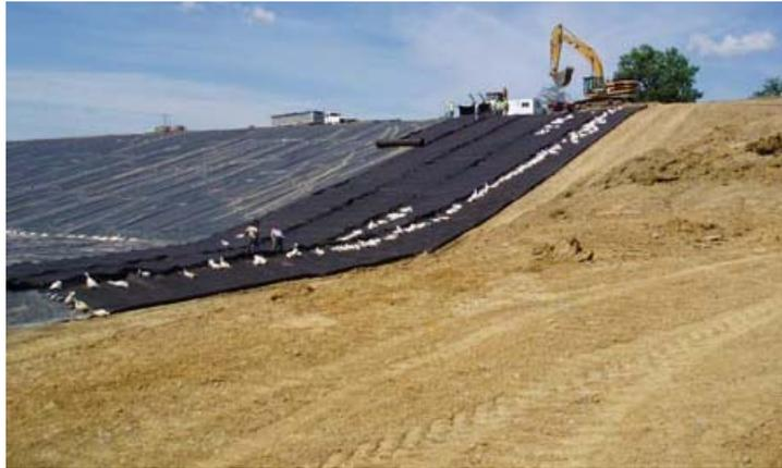
**Figure 2.4 - Winneshiek Co. Landfill Commission, Decorah. Cap cover construction stage of a landfill construction. ([www.jbholland.net](http://www.jbholland.net))**
