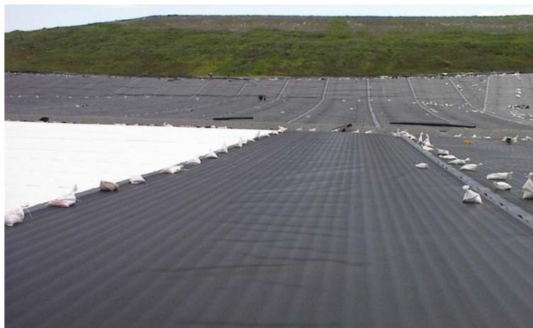
**Figure 2.6 – Geosynthetic liner of a landfill construction. ([www.cpengeers.com](http://www.cpengeers.com))**
