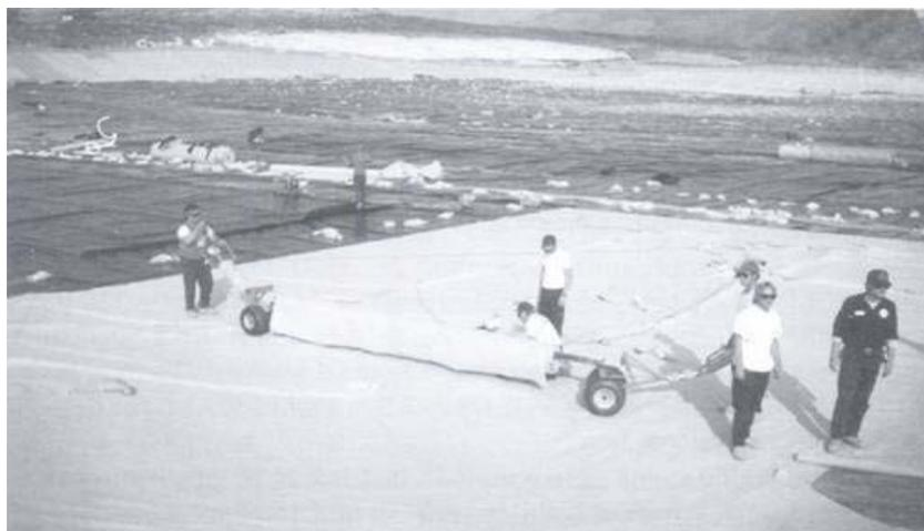
**Figure 3.2 – Pictures of GLS being installed (KOERNER, 1997)**
